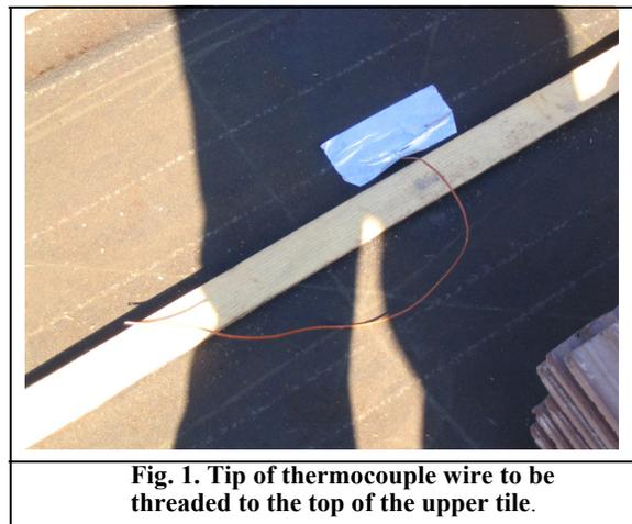
**Fig. 1. Tip of thermocouple wire to be threaded to the top of the upper tile.**
