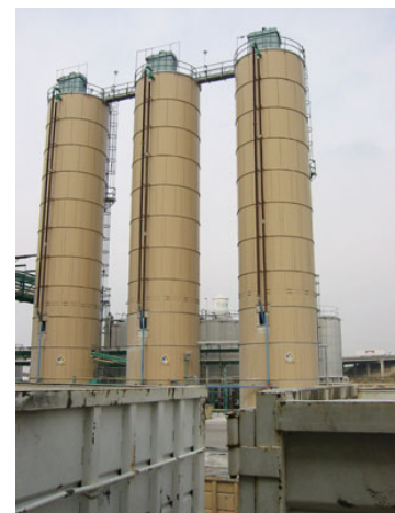
Figure 1. Granule silos at the Elk shingle plant in Shafter, CA.
