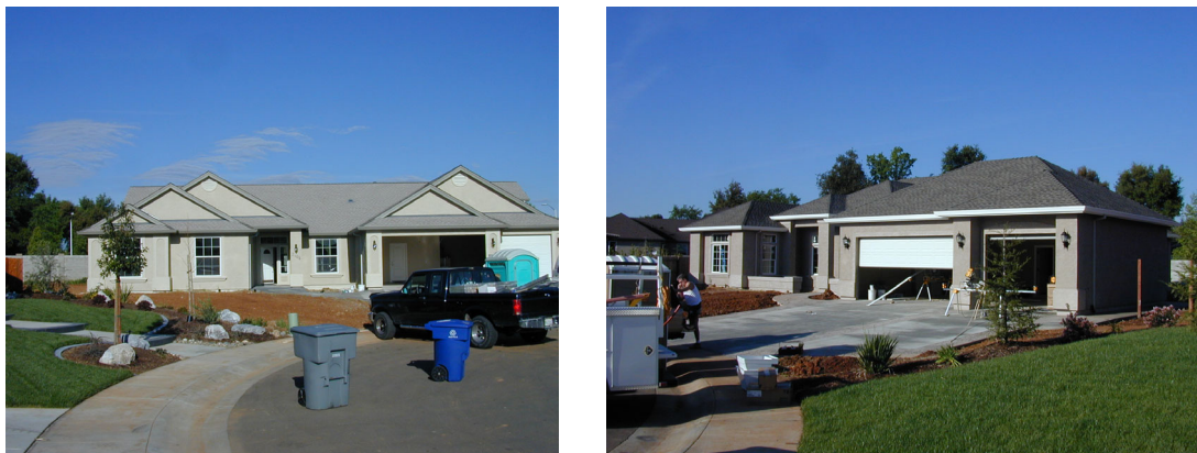
Figure 1. The pair of homes in Redding, CA demonstrating Elk's Weatherwood shingle having solar reflectance of 0.25 (left photo) and the conventional Weatherwood shingle having solar reflectance of 0.09 (right photo).
