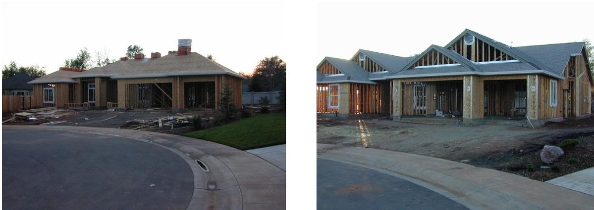
Figure 1. The pair of homes in Redding CA for demonstrating asphalt shingles with and without cool-colored coatings.
