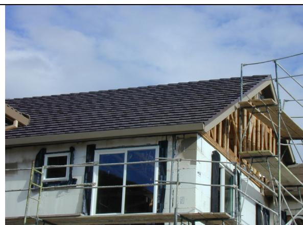
Fig. 2. Bustom-Bilt Metals ultra-cool metal shake was installed on the fourth demonstration house in Cavalli Hills.
