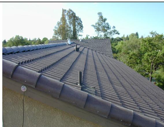
Fig. 3. Concrete tile roof with cool-colored coating from American Roof Tile Coatings.
