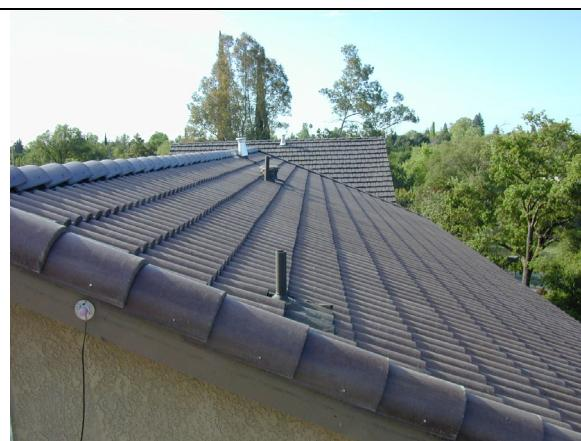
Fig. 3. Concrete tile roof with cool-colored coating from American Roof Tile Coatings.
