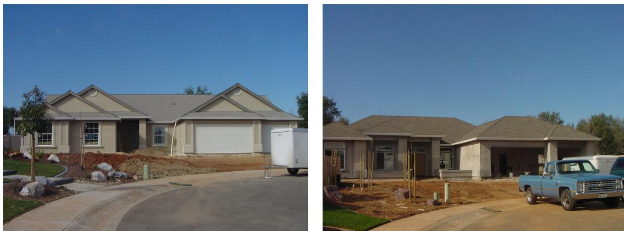
Figure 1. The pair of homes in Redding CA for demonstrating asphalt shingles with and without cool colored coatings.
