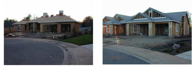
Figure 1. The pair of homes in Redding CA for demonstrating asphalt shingles with and without cool-colored coatings.
